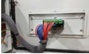
Numbered panel wires
