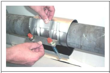
Step 2 Hook the bridge into the gap at the side bars.
