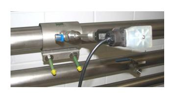
Example: Volume flow and consumption measurement
