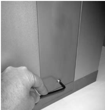
2. Remove single retaining screw.
